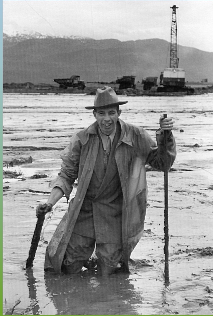
Charlie Ripley testing the dredged fill for the preload at the Alcan aluminum smelter in Kitimat April 1952.
